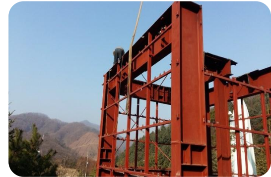
Iron structure building
