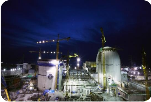
Nuclear power plant
