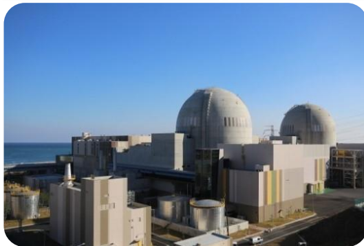
Nuclear power plant
