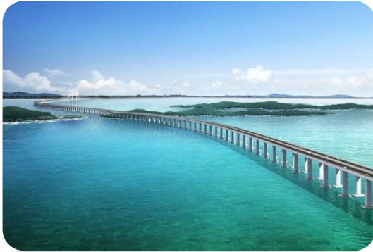
Steel structure bridge
