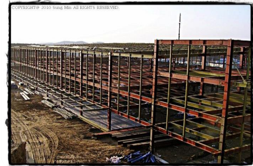
Iron structure building
