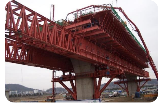
Iron structure building
