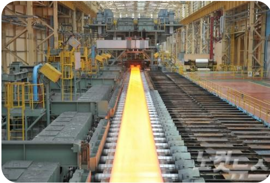
Iron & Steel plant
