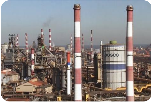
Iron & Steel plant
