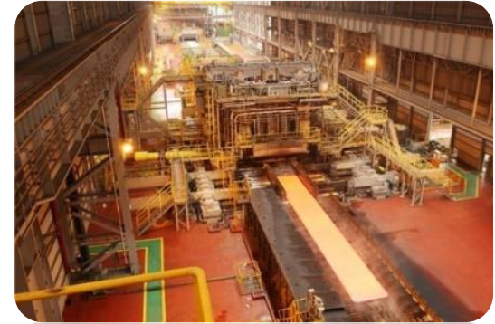
Iron & Steel plant
