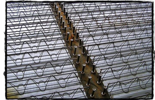
Iron structure building
