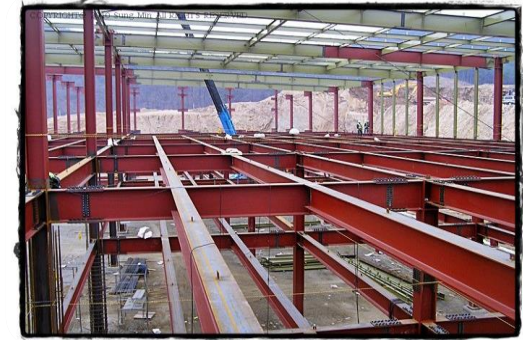
Iron structure building
