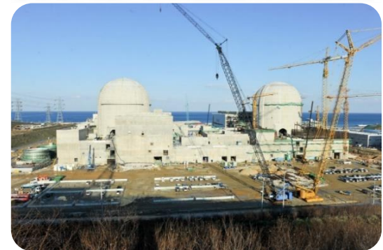
Nuclear power plant
