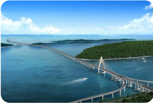
Steel structure bridge
