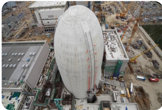
Nuclear power plant
